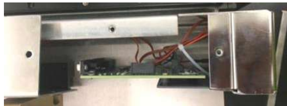
Figure A-9: Tying down the excess cable
